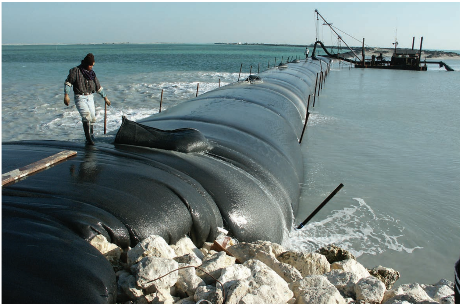
Infrastructure projects ensure a healthy demand for geotextiles worldwide. Courtesy TenCate
