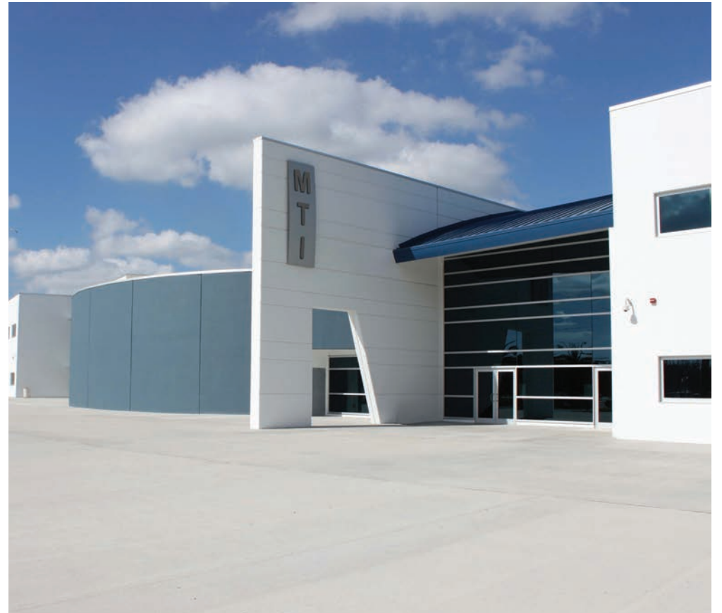
MTI recently renovated its offices
