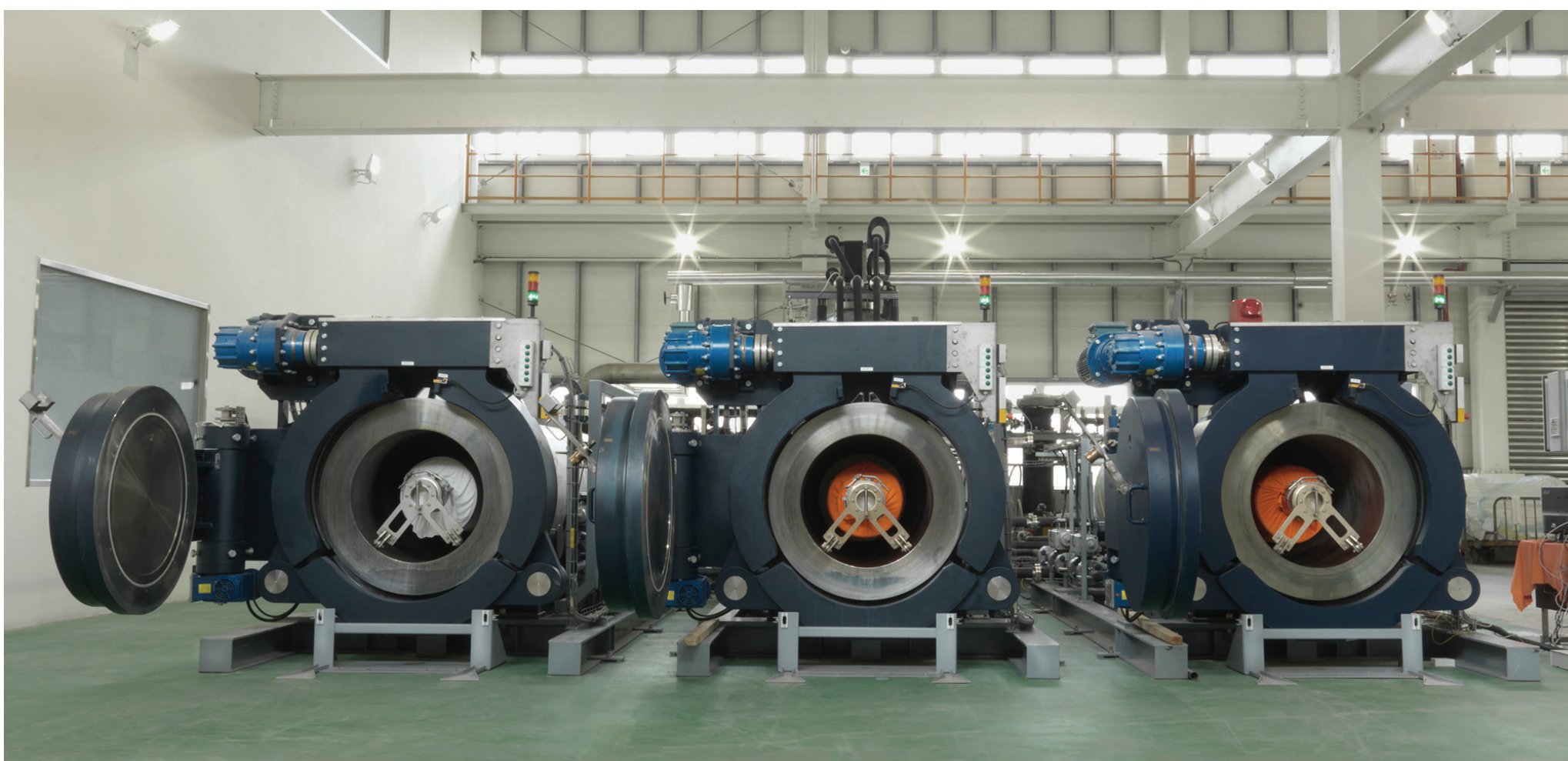
DyeCoo's technology consists of three vessels
